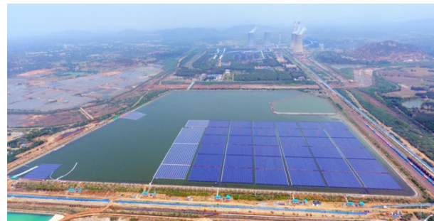
Fig. 1. Typical Floating Reservoir Solar Power Generation
